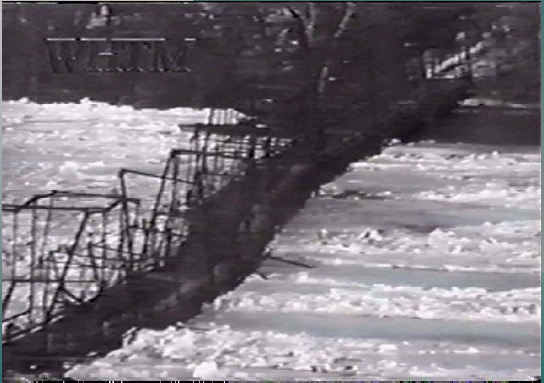
Walnut Street Bridge (Harrisburg, PA) collapse--January 1996
